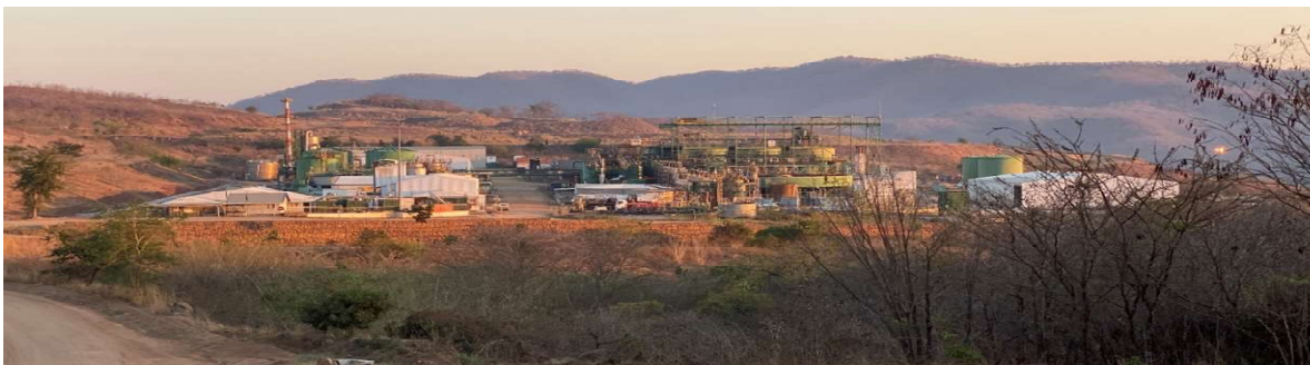
Figure 2: Kayelekera Process Plant and Surrounds – October 2019
